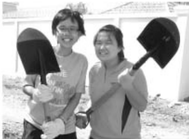
Road filling project.
